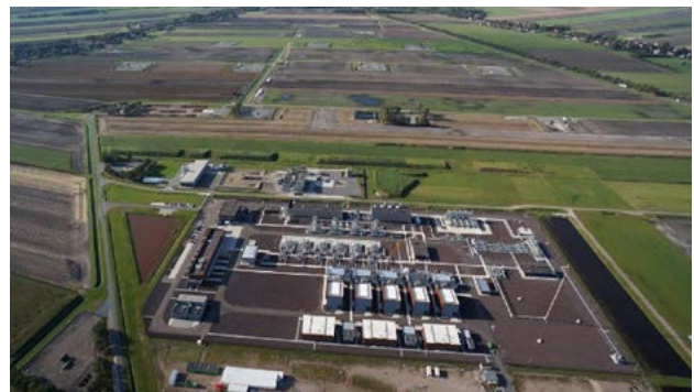
Hydrogen storage in salt caverns near Zuidwending
