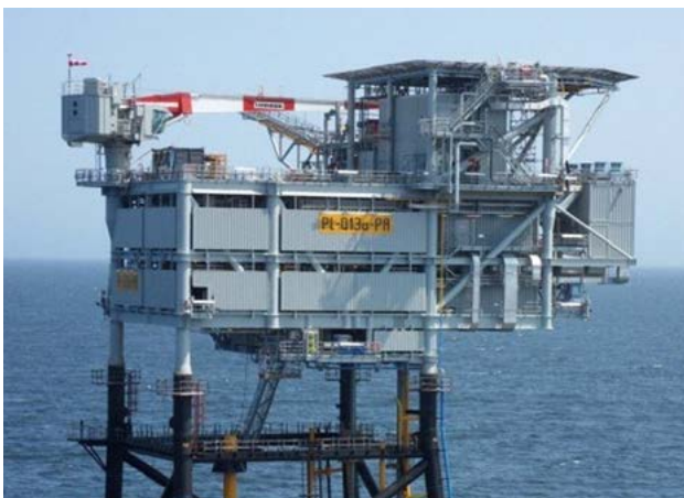
Neptune Energy platform Q13a in the North Sea, 13 kilometres off the coast of Scheveningen
