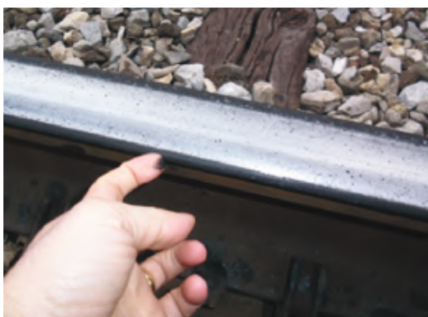
Figure 5: (Left): 48" grease dispensing bar attached to the inside of track to deliver grease to the wheel flange of rail car; (Right): Shows the presence of rail curve grease on the track wheel point of interface
